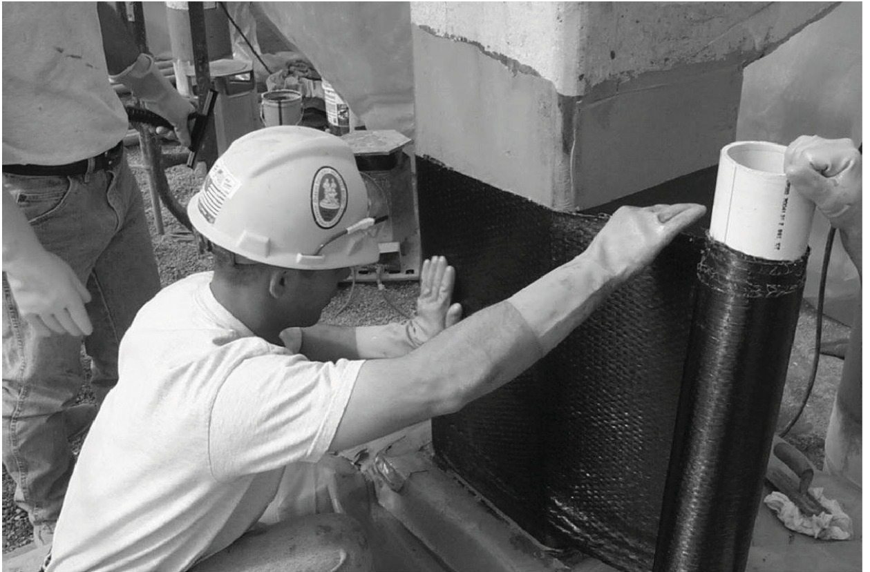
Figure 2.1a Installation of FRP wrap. (Courtesy of Sika Corporation.)
