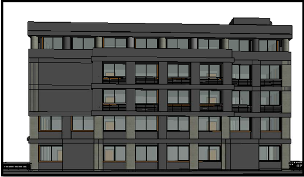
Photo 2: building (GS) north side view
