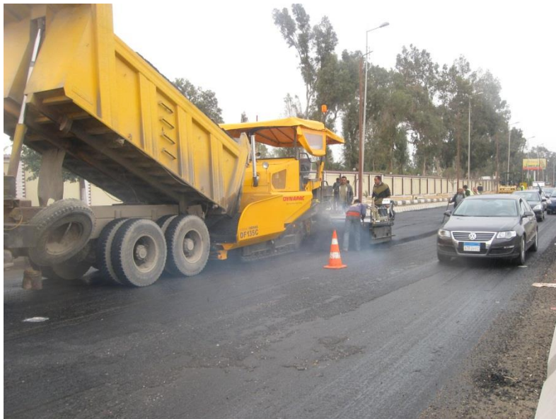
Figure 5.16 Placing of HMA by day
