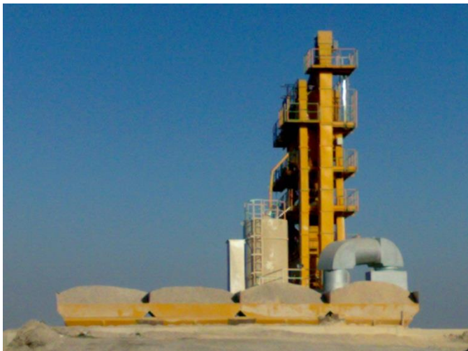
Figure 5.12 Kattameya Asphalt Mixing Plant (3)
