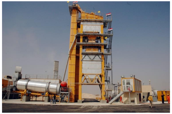
Figure 5.11 Kattameya Asphalt Mixing Plant (2)
