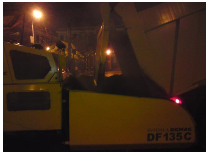
Figure 5.17 Placing of HMA by night
