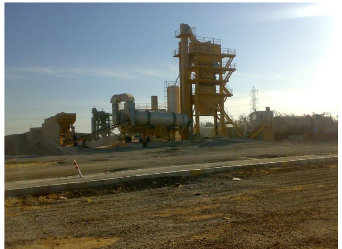
Figure 5.13 Kattameya Asphalt Mixing Plant (4)
