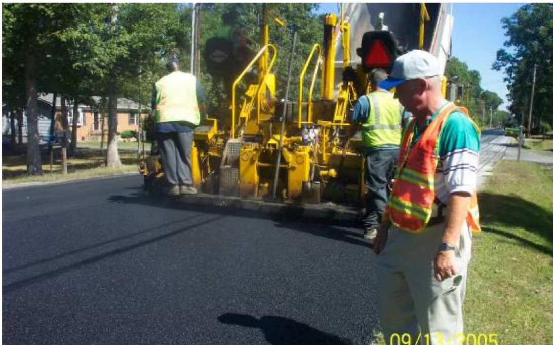
Figure 4.7: Surface course mix with Sasobit wax.
