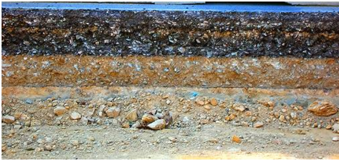
Figure 2.8 Asphalt Pavement Layers (1)
