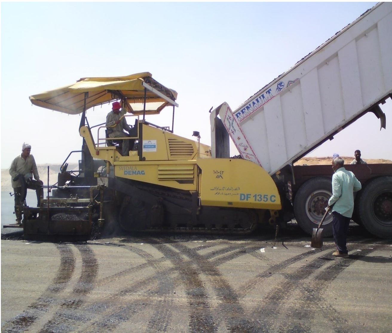
Figure 2.4 Asphalt paver fed by a dump truck
