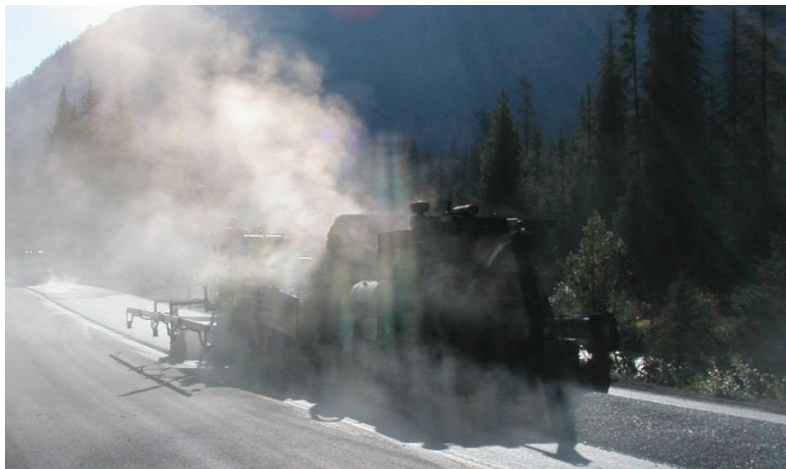
Figure 2.10 Showing Asphalt Emissions during Placing
