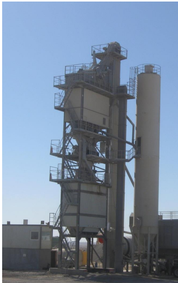
Figure 5.3 the New Runway Project (Cairo International Airport) Asphalt Plant
