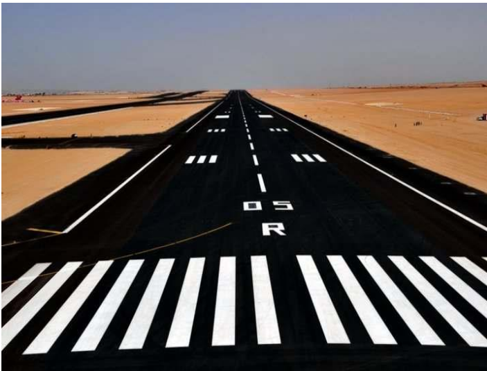
Figure 5.1 the New Runway Project (North) (Cairo International Airport)
