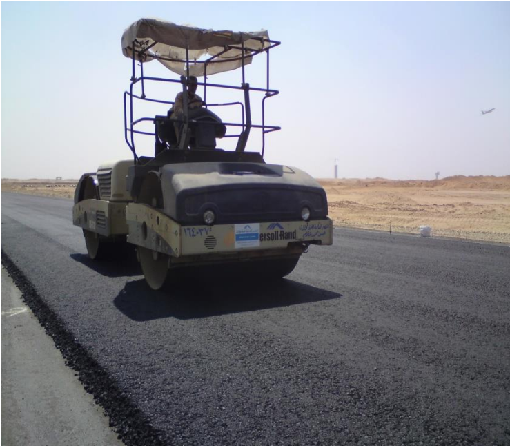
Figure 2.5 Vibratory Roller Compactor
