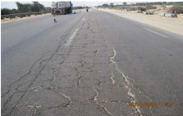
Figure (3.2) Cairo/Alexandria freeway cracks
