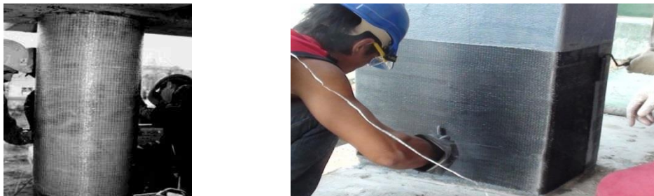
Fig. 3-5 - Wrapping columns with FRP
