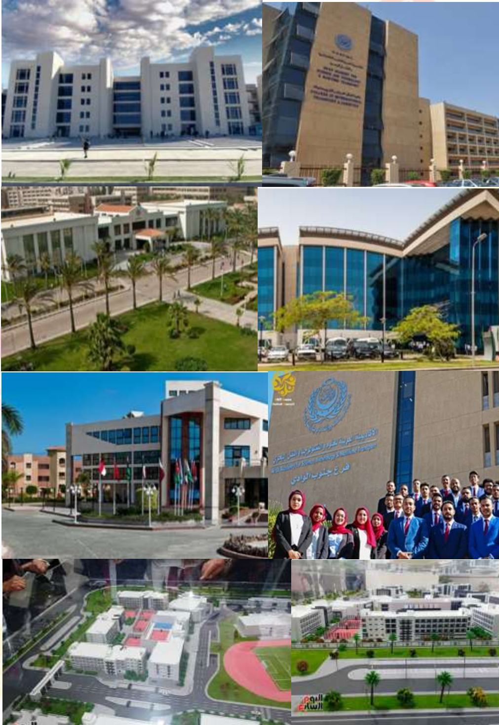
Building on brownfield sites on AAST webpage
