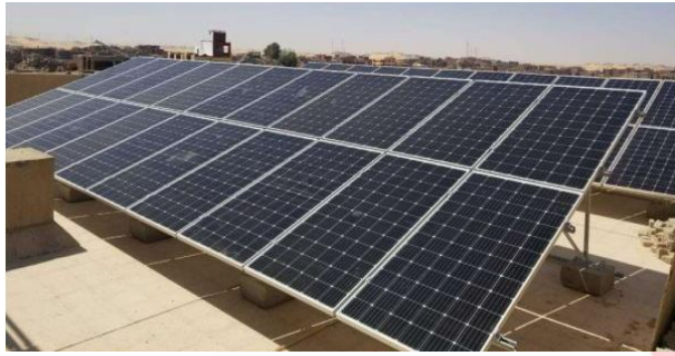
Figure 1. 150kW solar power station in Aswan campus
