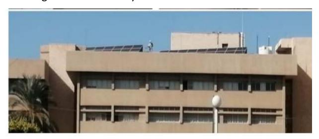
• 50 kW Solar Power Plant (On-Grid) with Weather Station. Installed on floor of building G.
