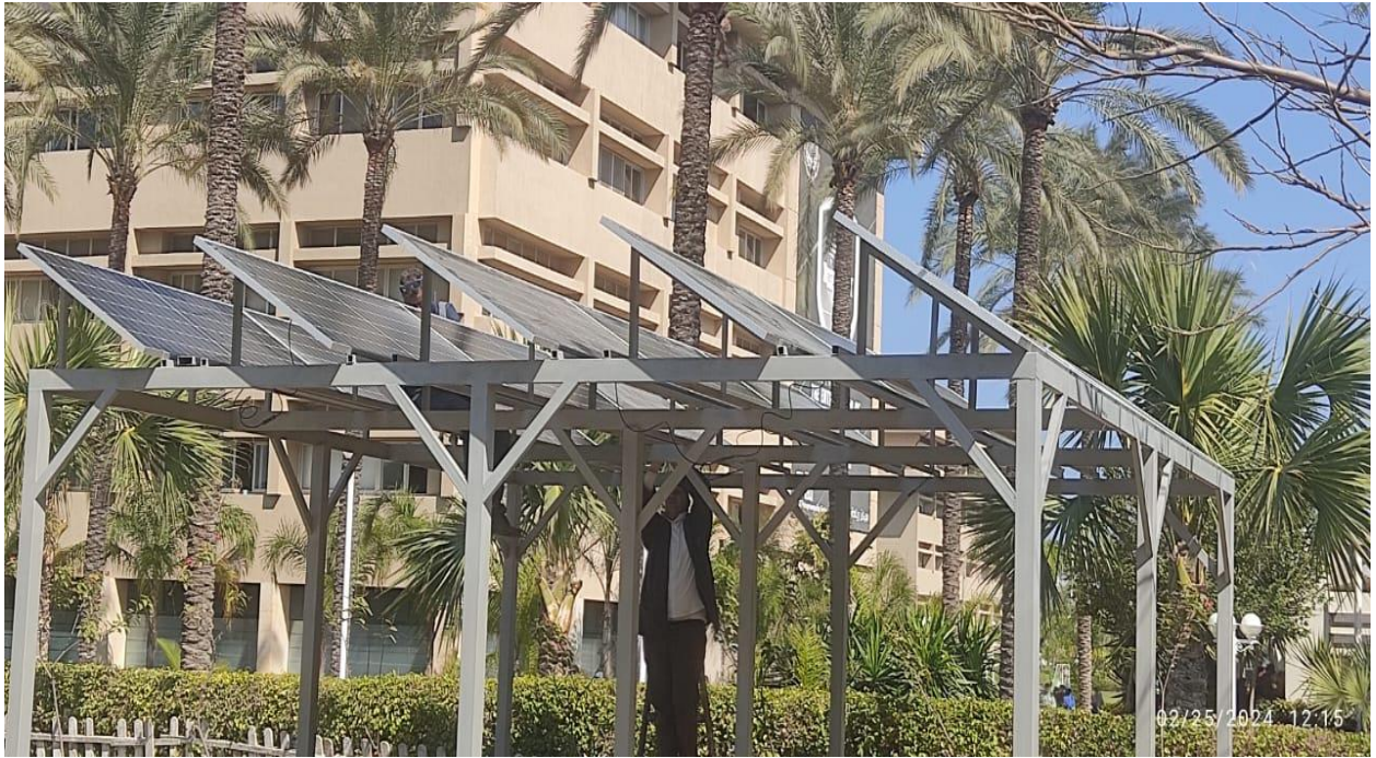
Figure 3: Solar PV Modules Mounting Structure
