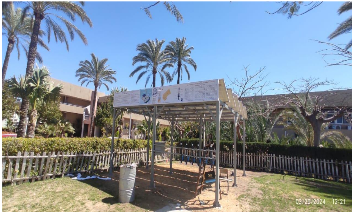
Figure 3: Solar PV Modules Mounting Structure
