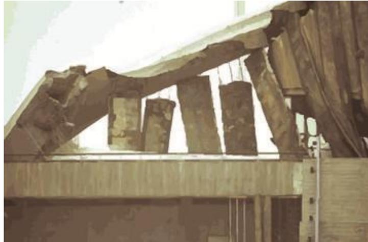
**Fig. 1.1:** Close up view of collapsed beams, Berlin Congress Hall
