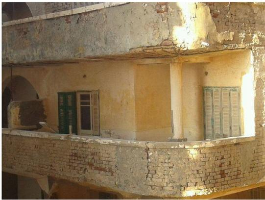
**Fig. 1.5:** Concrete cover spalling, Alexandria, Egypt
