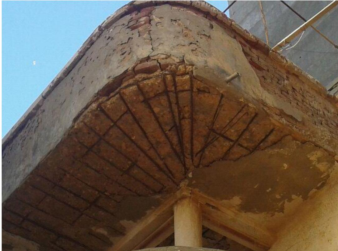
**Fig. 1.7:** Total concrete cover spalling and exposure of the reinforcement to direct corrosion, Alexandria, Egypt
