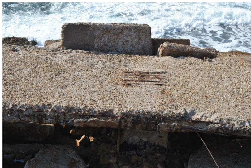
**Fig. 3.15:** Abrasion & cement decomposition in tidal zone
