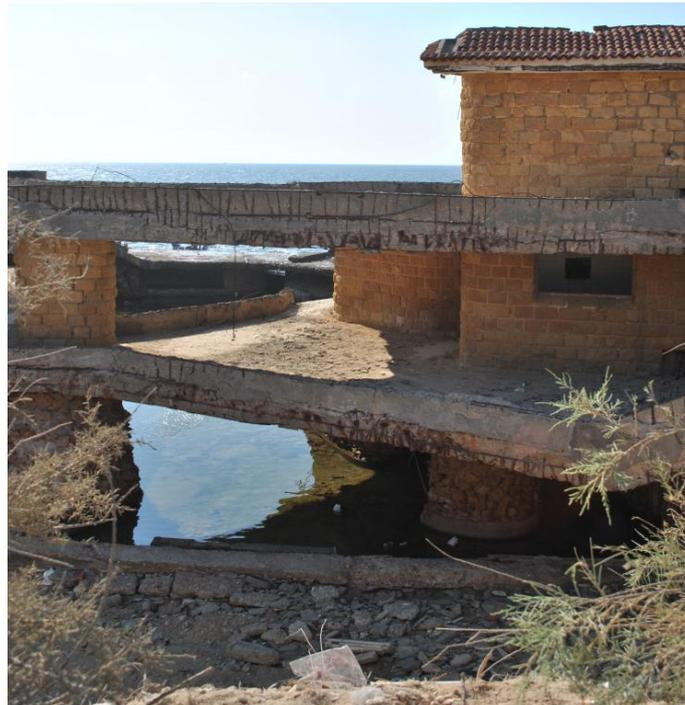
**Fig. 3.14:** Concrete cover spalling
