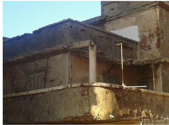
**Fig. 1.6:** Deterioration of building's frontage, Alexandria, Egypt
